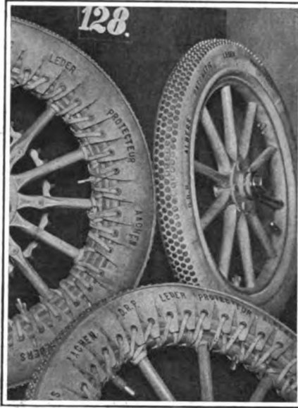
TIRE PROTECTOR AND ANTI-SKID.
